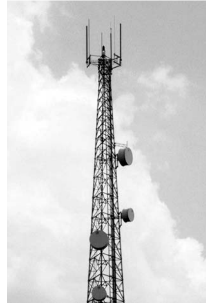
Tower with RFS Omni Antennas
