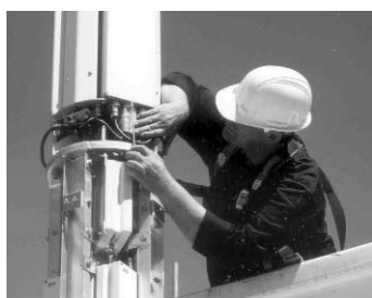
Attaching optional Optimizer RT remote tilt units
